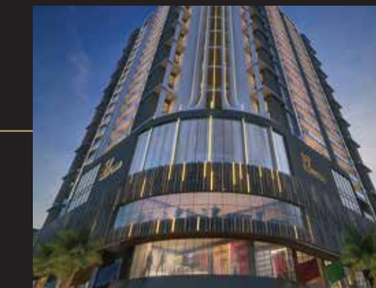
57 MIDTOWN COMMERCIAL SHOPS & SHOWROOMS WAKAD
